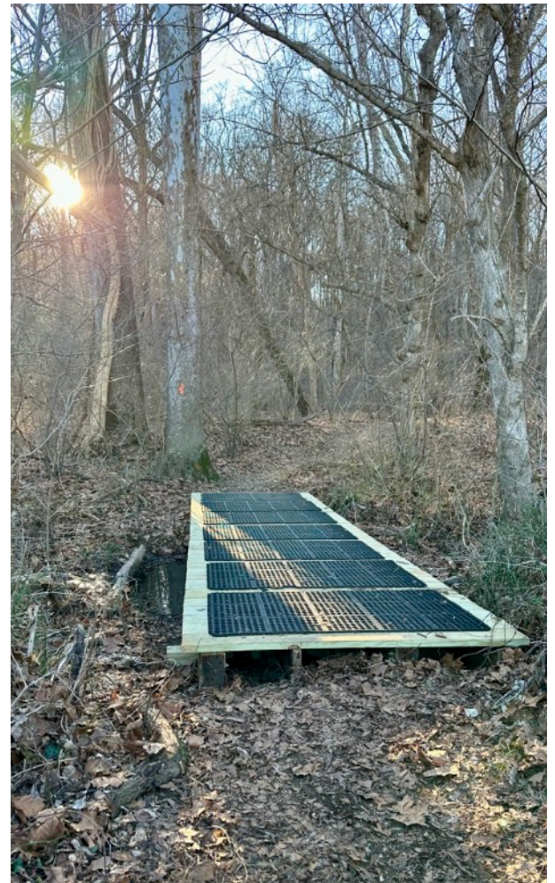
The finished bridge
